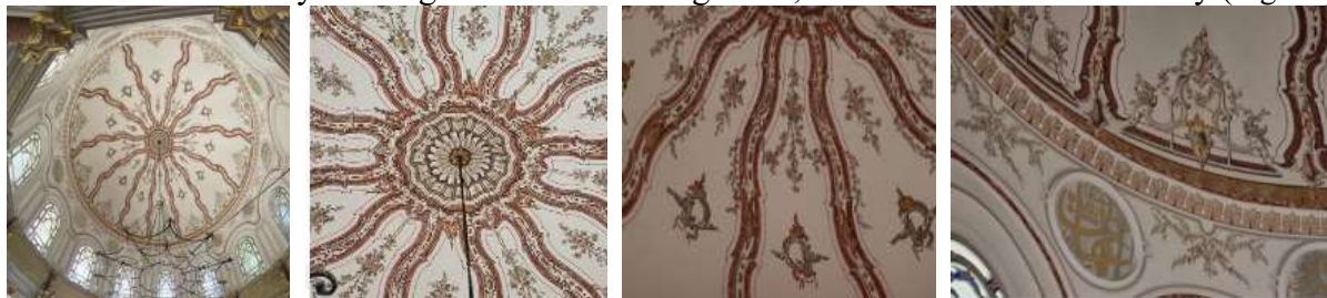
Figure 54: Central dome of the Mihrişah Valide Sultan Tomb © The researcher ; Figure 55: A detail of the dome's decorations © Bodur 2024 ; Figure 56: A detail of the dome's decorations © Gürlek 2019 ; Figure 57: A detail of the dome's decorations © Ürkmez 2025.
