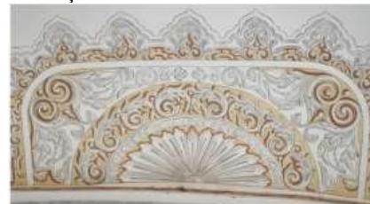
Figure 43: Dome's decorations, the rewaq of the Mihrişah Valide Sultan Tomb © Ürkmez.
