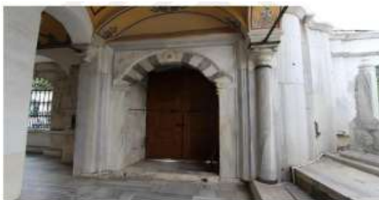
Figure 16: The door opening in the front façade © The researcher.
