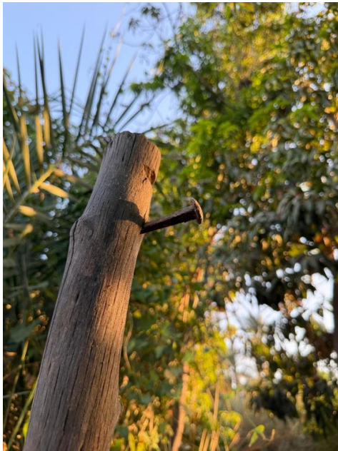
Figure 18: detail of the top of the counterweight pole with the metal nail, by the author (March 2026).
