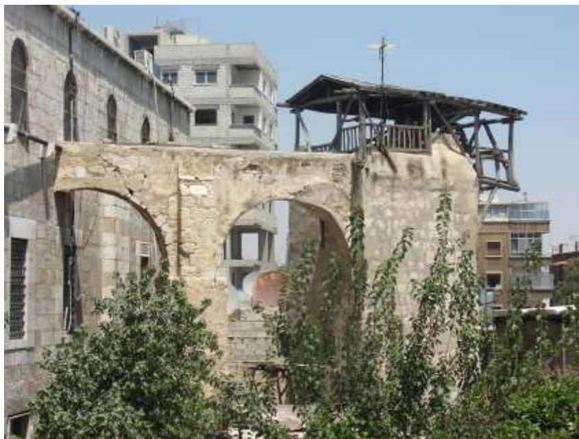
Figure 12: General view of the waterwheel and channel connected to the Muhyiddin Ibn Arabi Mosque. © Author's Collection
